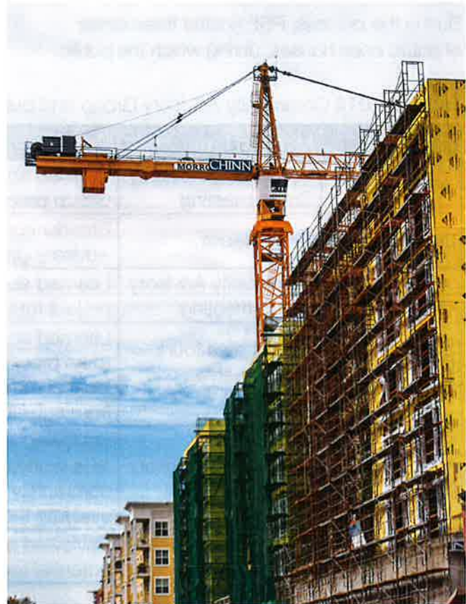
Construction in Redmond
